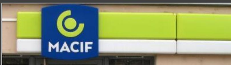
Coquille MACIF, PMMA frost 4 mm
